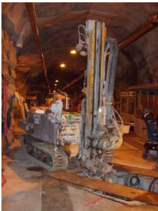
Figure 3. a) The drilling rig placed over the deposition hole. b) Cores taken form the buffer (Johannesson 2007).
